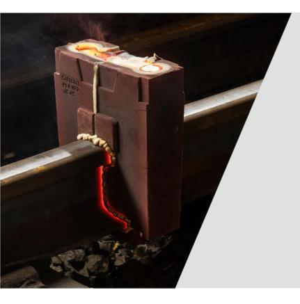
Pandrol's AutoSeal® – the world's first self-sealing mould – significantly streamlines the aluminothermic welding process.
