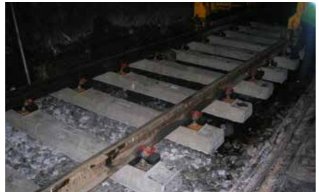
Installation on ballasted track.
