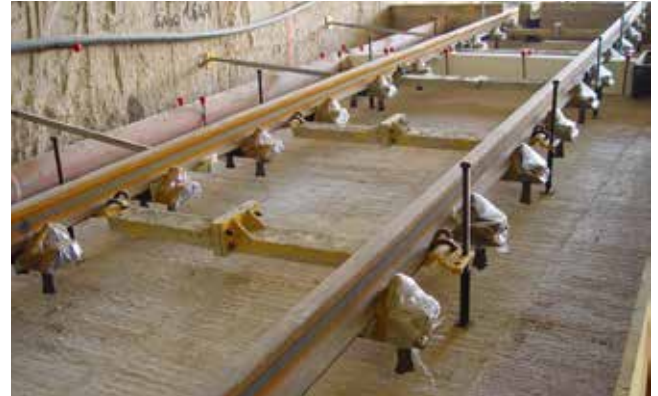
Top-down DFF installation.
